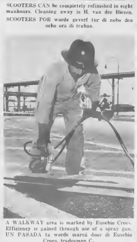
A WALKWAY area is marked by Eusebio Croes. Efficiency is gained through use of a spray gun. UN PANADA ta wordé marcaá door di Eusebio Croes, tradesman C.
